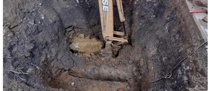
*PHOTOS ATTACHED: Left: AWA crews work through the night Labor Day weekend to repair a breach in the major pipeline supplying untreated water to Ione. Right: The exposed section of the 16-inch iron pipeline showed significant corrosion and the miles-long Ione Transmission Line is now scheduled for priority inspections and testing to determine the overall condition of the 35-year old pipeline.*
